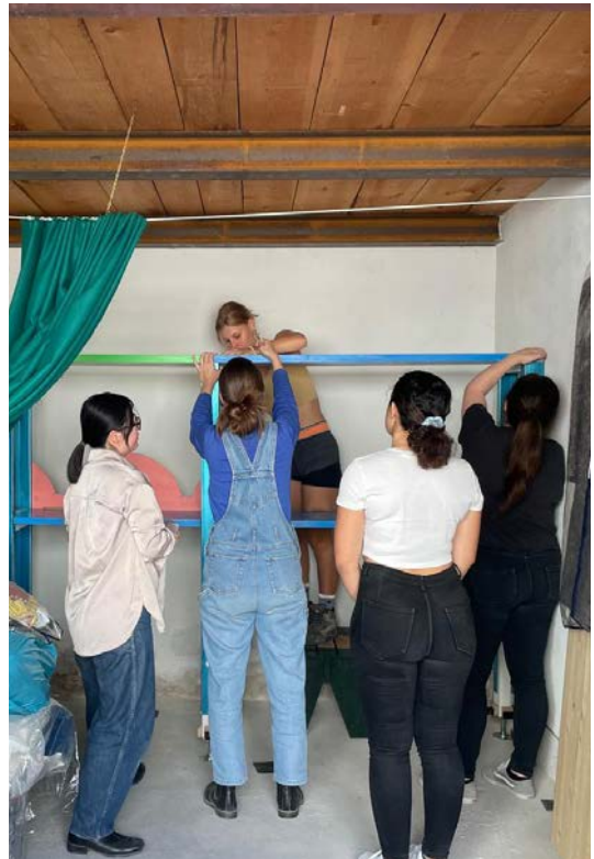
construction on site
